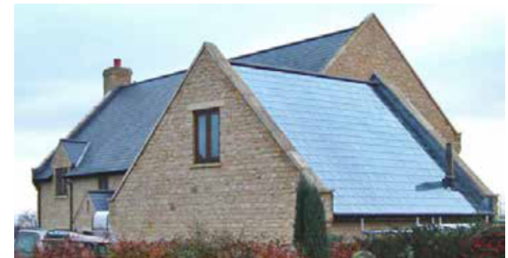
Figure 84: Integrated design for solar panels.
