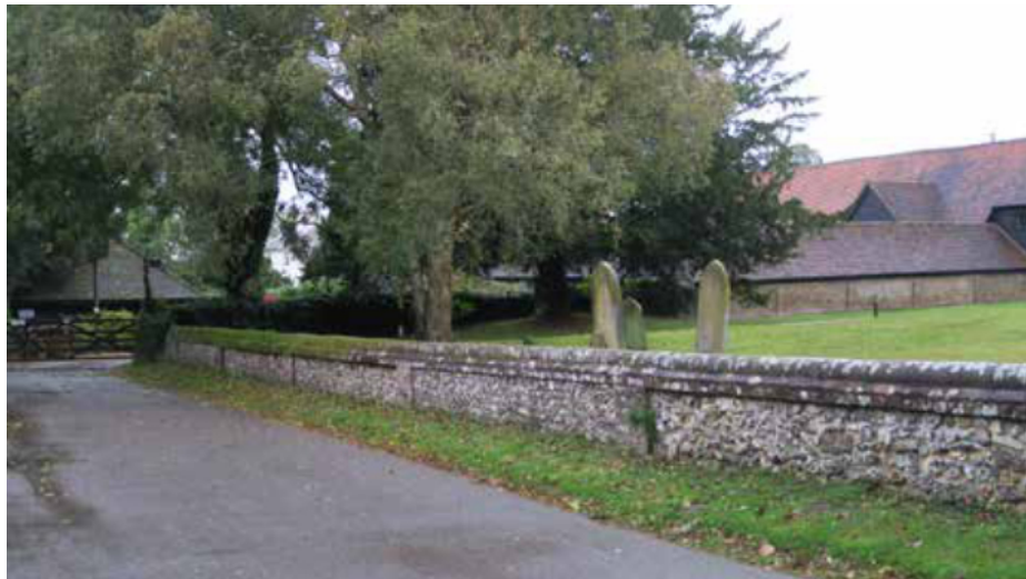
Figure 72: Church yard wall built with local flint.
